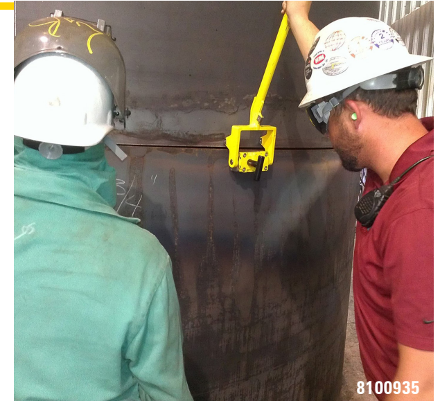
Sheet Alignment with MagPress
